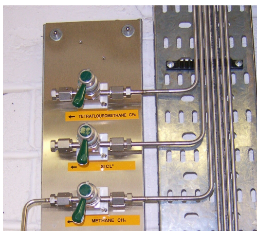
Figure 13 Gas supply point-of-use valves
